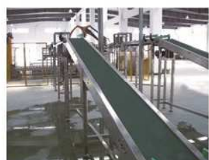
Inclined conveyor in steel steel frames
