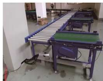
25. Interflow line with belt and roller c/v
