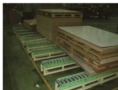
Gravity roller sections as moving tracks for pallets
