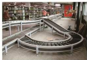
21. Leveled conveyor system in storehouse
