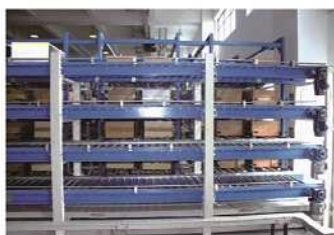
23. Leveled roller c/v lines in warehouse
