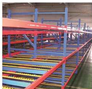
Racks with flow rails
