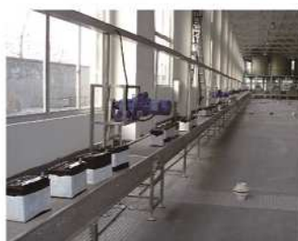
26. Storage battery unit delivery line
