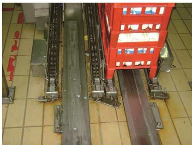
Full stainless steel application with turnover boxes directly on the conveyor
