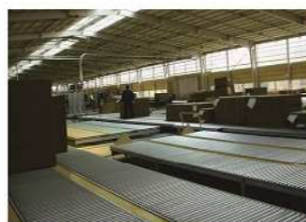
18. Gravity ground roller conveyor lines
