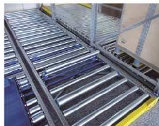
30. Pallet delivery in racking systems
