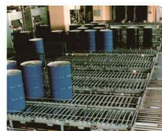
28. Roller conveyor line for oil cans
