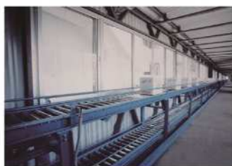
22. Leveled roller c/v delivery line
