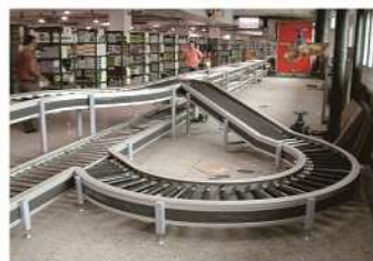
21. Leveled conveyor system in storehouse
