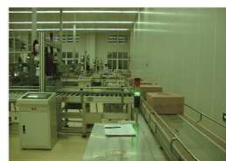
12. Cartons distribution with slat chain conveyors
