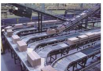
10. Cartons delivery system with interflows
