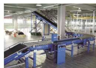
16. Delivery line between floors
